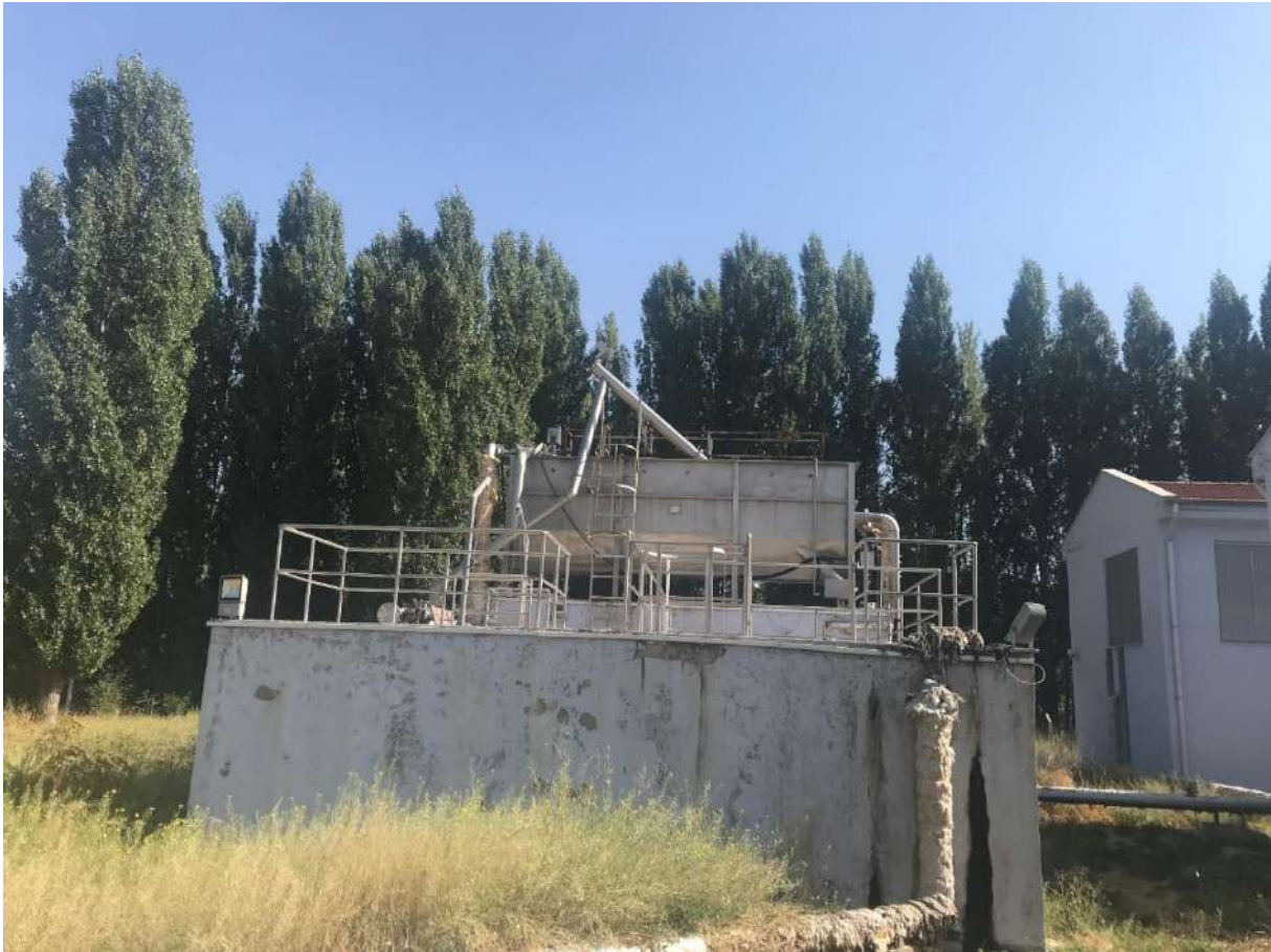
Figure 58. Images from NOHU Sewerage Waste Disposal-2
