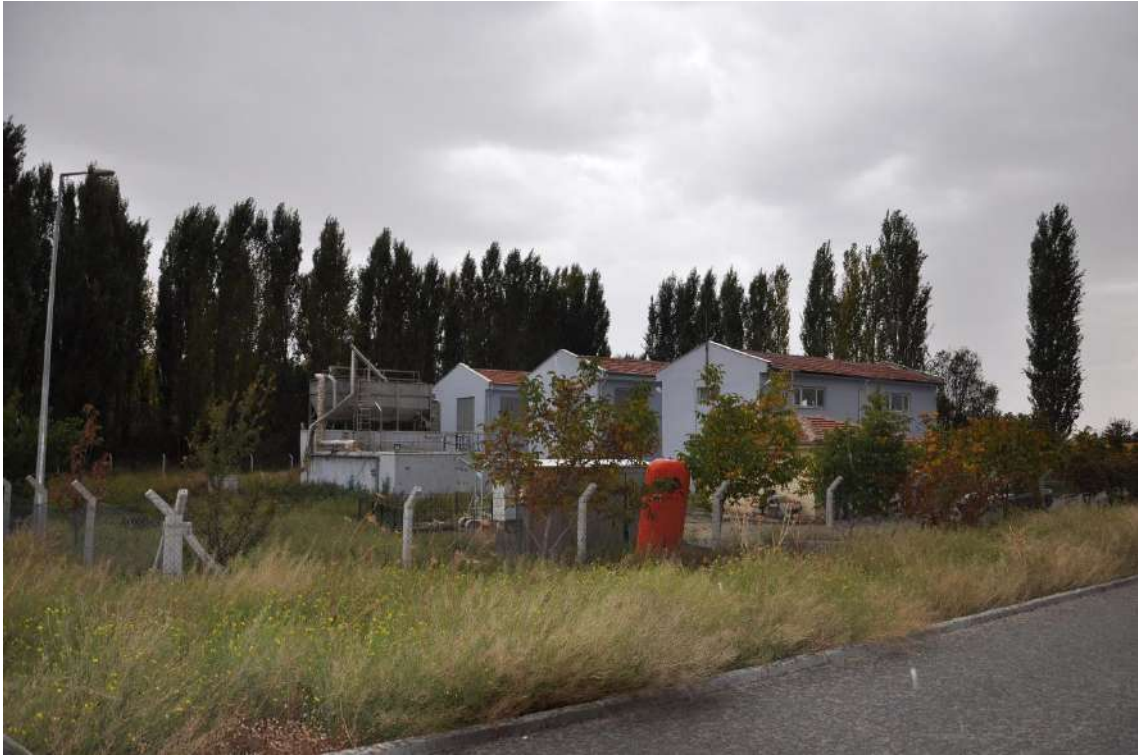
Figure 57. Images from NOHU Sewerage Waste Disposal-1
